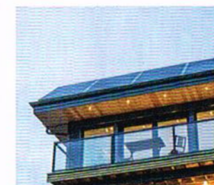
Straka's rooftop garden (above) is a labour of love that will never recoup its cost. By contrast, the solar panels (visible above and at right) are designed to provide a return on investment. Straka calculates that by selling electricity to the Ontario Power Authority, the solar system will break even in seven or eight years.
