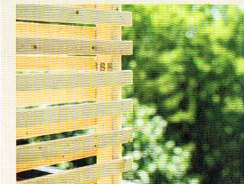
Two years after moving in, Straka is finally finding time to finish the details, including green canopies over the porches (to keep the indoors cooler) and these "walls" between the two houses on each balcony. The slatted walls are designed to allow both air flow and privacy.
